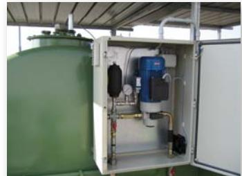
Includes a bypass valve preset on 28 bar pressure.
